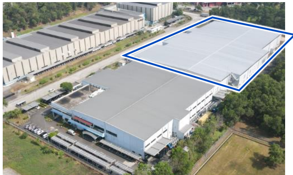
▲PT. SIIX EMS INDONESIA in Jakarta Construction of the second building completed (Sep. 2021)
