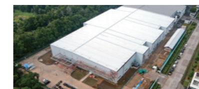
Second building of Karawang Factory in Indonesia under construction
